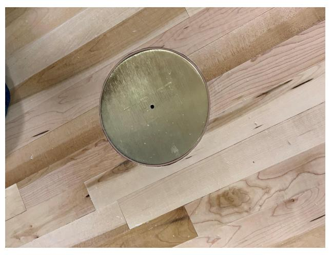
A few weeks ago I detailed the steps in installing the gym floor. I mentioned the bolts holding the subfloor to the concrete did not have threads and were simply driven into holes drilled into the concrete. This is one of those bolts. Notice the hump and also notice the rubber washer at the head of the bolt. It is very simple and it works.
