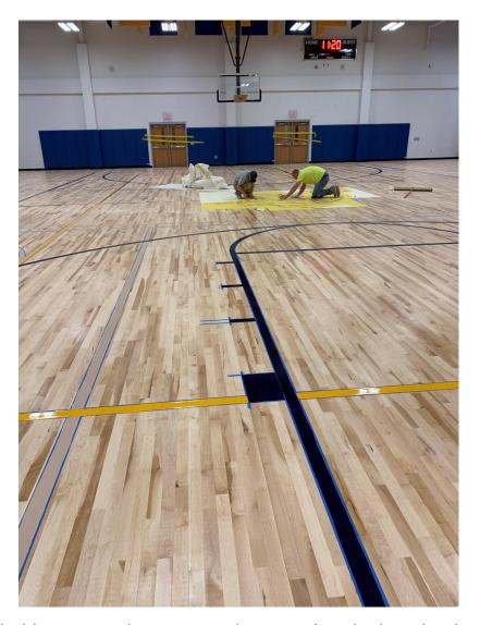
The light blue narrow lines you might notice beside the other lines is the tape used to mark the edge of the painted line. Painting the lines is a "simple" matter of painting between the two tape borders. It sounds so easy!
